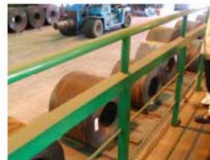
Fig.1 Handrail in the factory
